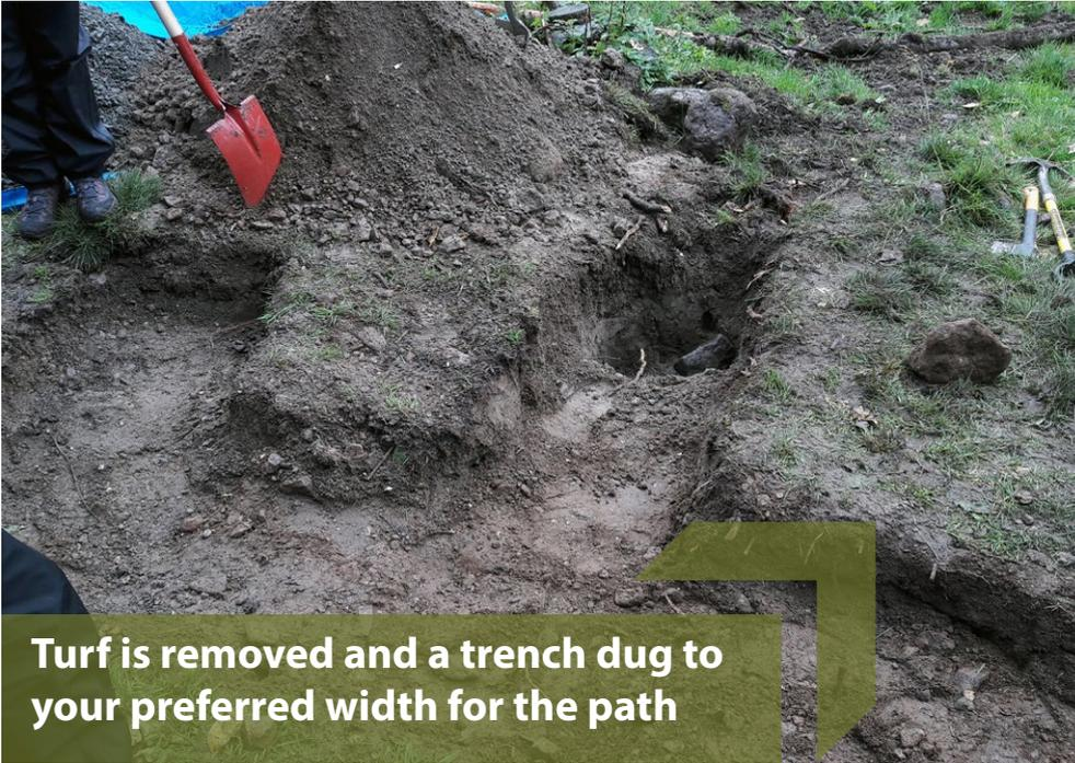
**Turf is removed and a trench dug to your preferred width for the path**
