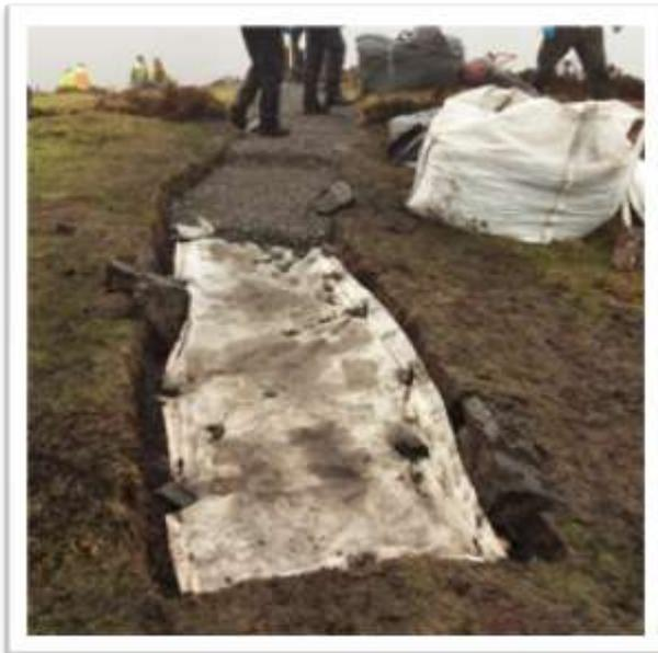
*Figure 16 - Aggregate path on suitable gradient.*
